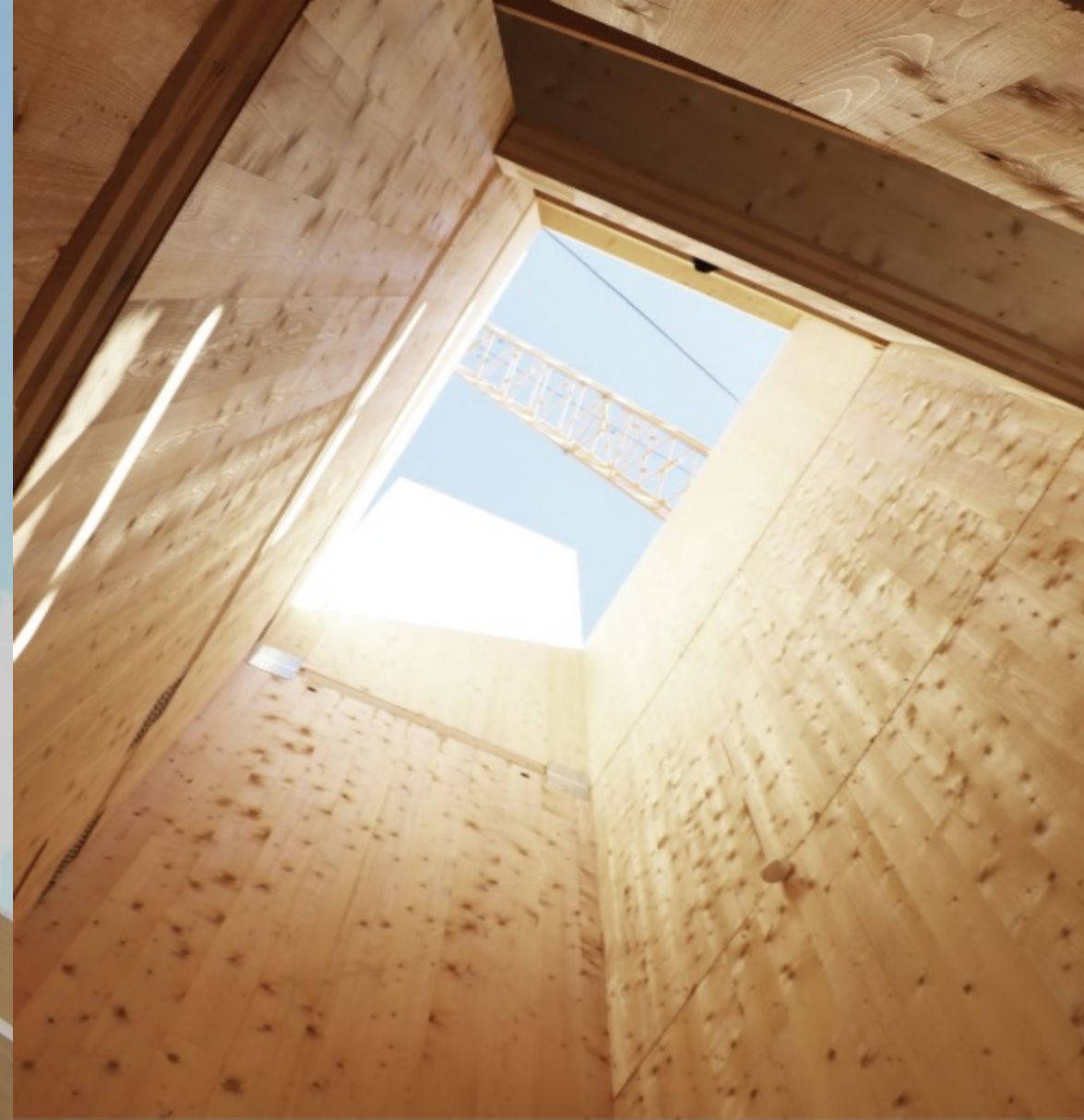
• CLT to elevator shaft
